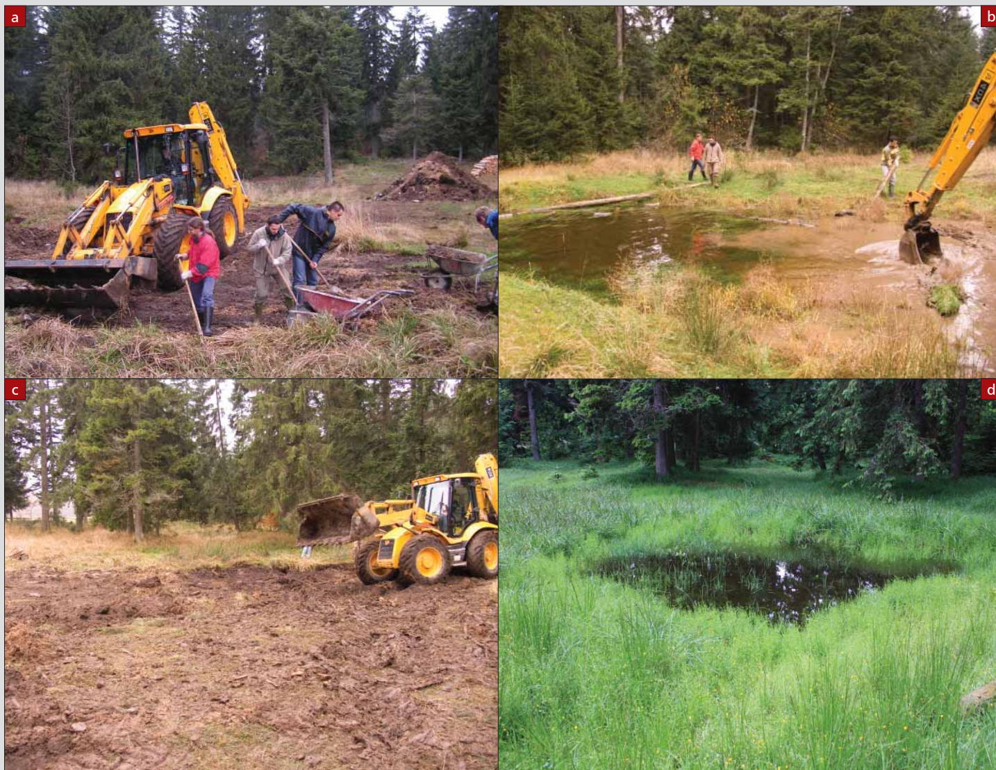
Figure 35. a), b) and c) the restoration of two ponds in Sunger in late 2008, d) the other renovated pool during the summer of 2010 (PHOTO BY DUŠAN JELIĆ AND MARKO PEČAREVIĆ)
